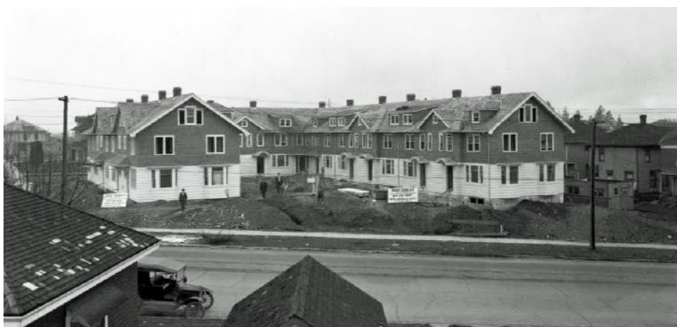
GRAY GABLES UNDER CONSTRUCTION C. 1922
